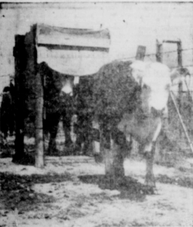
SELF-SERVICE SPRAYING STALL—Agriculture experts of the University of Illinois suggest up this bovine "beauty parlor" at Dixon Spring, Ill., where fly-tortured cattle can get relief. When Dossie walks through the stall, the trips a bellows mechanism that releases insecticide over her body, killing pesky horseflies.
