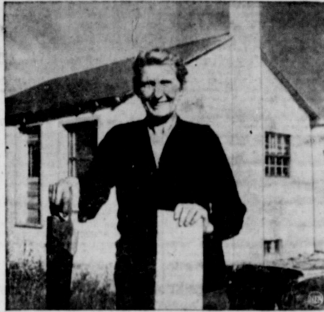
GRANDMA'S A "KRAFTS-MAN" —In Howell, Mich., everyone is talking about Mrs. Mary Kraft, 63-year-old grandmother, shown standing in front of her five-room house which she built by herself. The only help she received was in excavating for the basement when her 13 grandchildren pitched in, plus some finishing touches on the electric wiring and the top of the chimney. Mrs. Kraft is proudest of the fact that her house is only an inch off plumb at one corner. Next projects on her list are a front porch and breakfast nook furniture.
