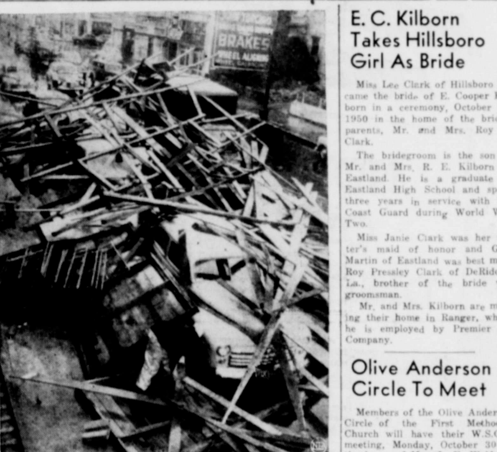
NORTHERN CALIFORNIA LASHED BY HIGH WINDS —Automobiles parked along Oakland Street in Oakland, Calif., are buried under wreckage of scaffold blown down during 42-mile-an-hour gale which lashed the bay area. (NEA Telephoto).
