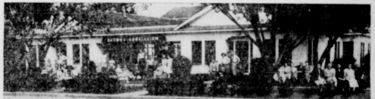
Front View of Sanatorium After Recent Remodeling and Enlarging
