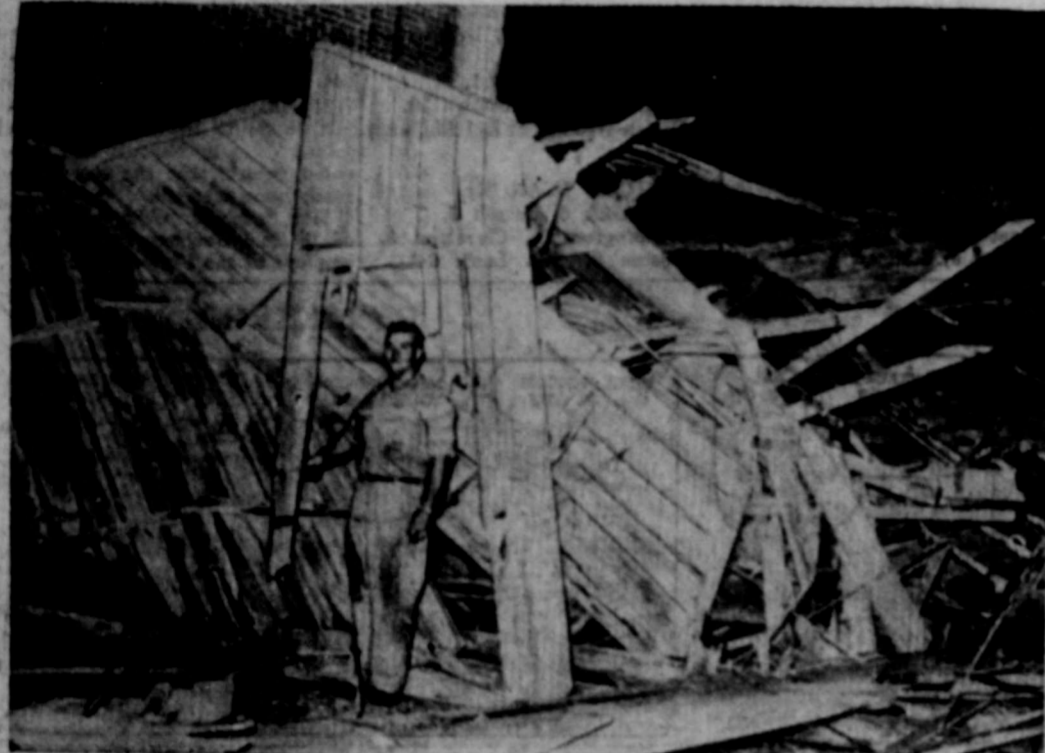
IN TEXAS TORNADO'S PATH —Tom Waugh stands by a demolished cooling tower at the Public Service Company's power plant, Perryton, Tex., after a mighty tornado ripped through the Texas panhandle. One person was killed and 13 others injured at Perryton during the storm. (NEA Telephoto).
