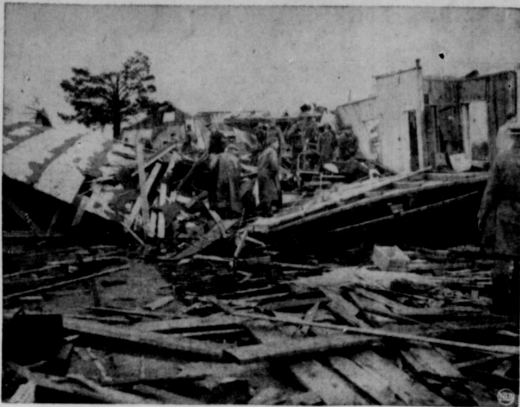
Rescue workers search thru the debris at Slack Air Base near Shreveport, Louisiana, following a tornado which hit shortly after noon. Had it struck earlier the loss of life would have been much greater. Three men were killed in this mess hall. (NEA Telephoto.)
