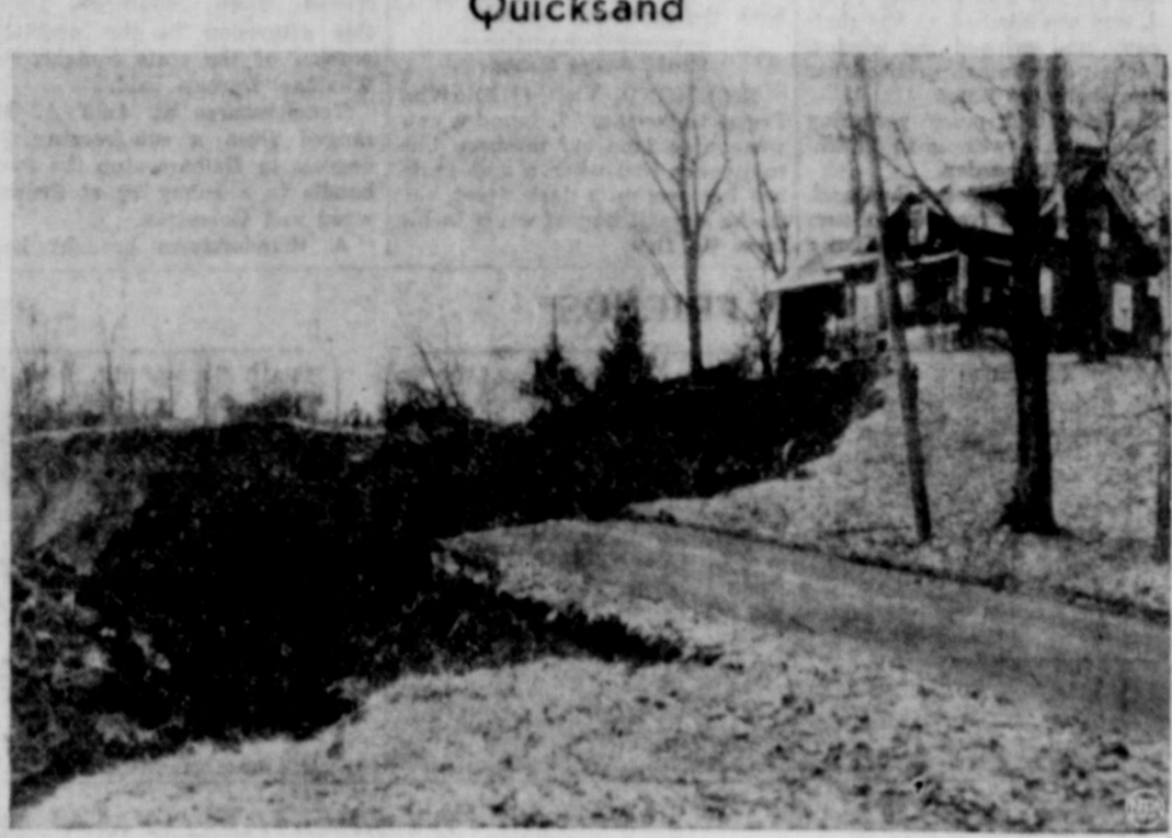
This house at Brecksville, Ohio, rested precariously on the edge of a huge crater after a freakish landslide wiped out 500 feet of road bed, ruined a State Highway Dept. building and buckled Baltimore and Ohio railway tracks. A family of four, asleep when the slide occurred, was aroused by the city water department employees who were working nearby. (NEA Telephoto.)
