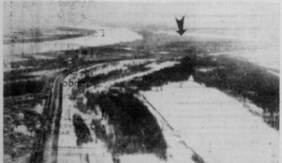
Looking to the south toward Cairo, Illinois (arrow), the Ohio river is at left and the Mississippi at right background. In the foreground is flooded lowland from which hundreds of families have been evacuated. Army engineers are considering breaking the levees in this vicinity to decrease the danger to Cairo. (NEA Telephoto.)
