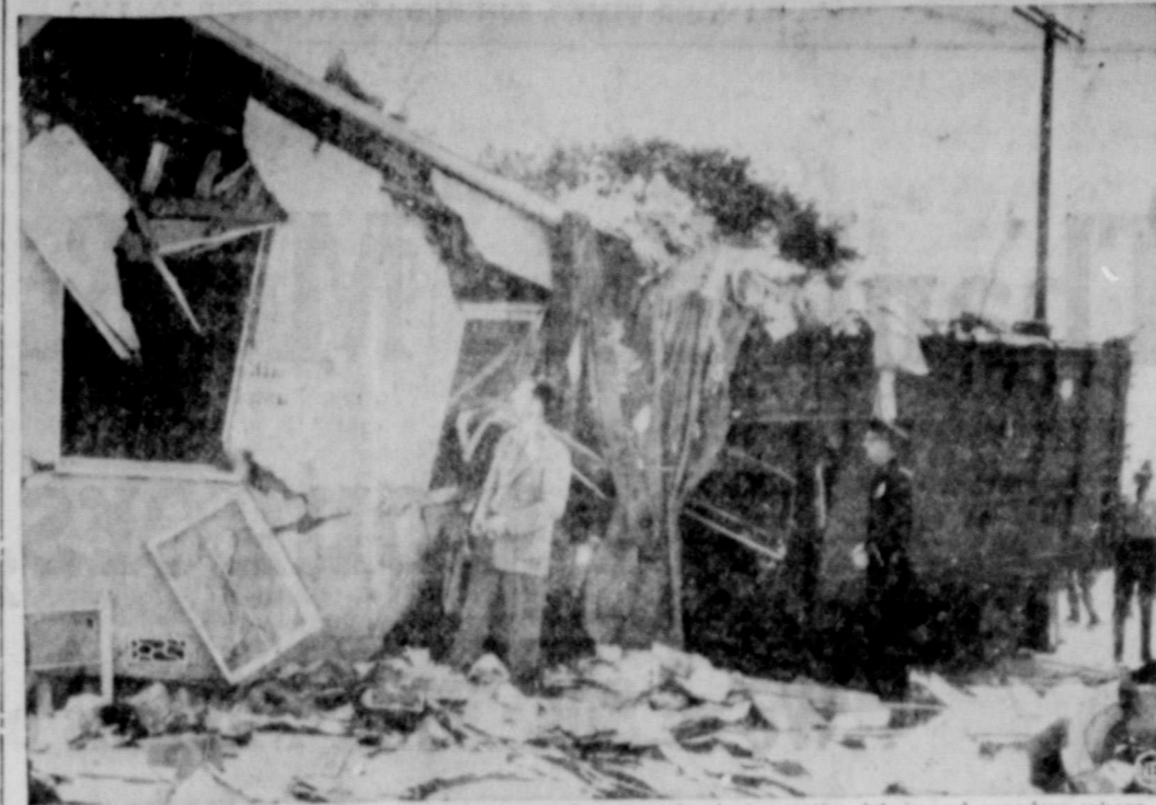
NO PLACE LIKE HOME —Bob Tolomei of Los Angeles looks at the debris and wonders where the wreckage of his home ends and the rubbish from the truck begins. The rubbish truck blew a tire, mowed down a lamp pole and completely rearranged the Tolomei home before coming to a halt. Occupants of the truck were hurt only slightly.
