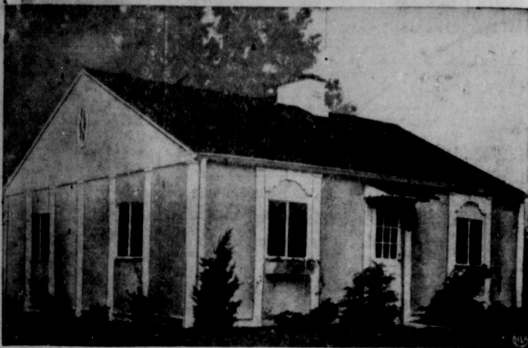
HOME FOR FAMILIES MAKING $40 A WEEK — The new four-room prefabricated home above is being built by a subsidiary of U. S. Steel to sell for $6300 or less, including a landscaped lot. Known as the "Champion," the low-cost house—designed for families making $35 to $40 a week—is being turned out by Gunnison Homes, Inc., at New Albany, Ind. Before long, it will be available in all sections of the country. The house is built largely of plywood. Features include forced air heating system, complete insulation and streamlined kitchen. Varied exterior designs will avoid "sameness" when the houses are built in groups. Prices will vary according to location, but the "Champion" is designed to sell for a down payment of as little as $350, and monthly payments at about $37.
