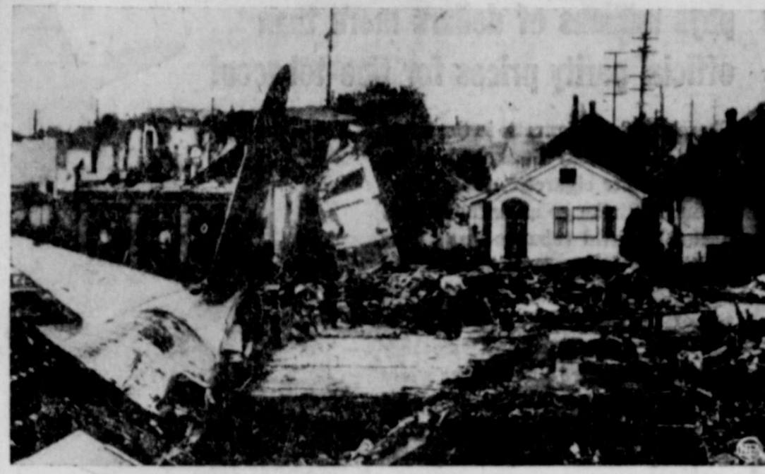
A C-46 attempting to take off from Boeing Field, Seattle, Wash., struck a power line and crashed into homes adjoining the field. Six occupants of the homes were killed. Three of the 32 persons aboard the plane are missing. (NEA Telephoto.)
