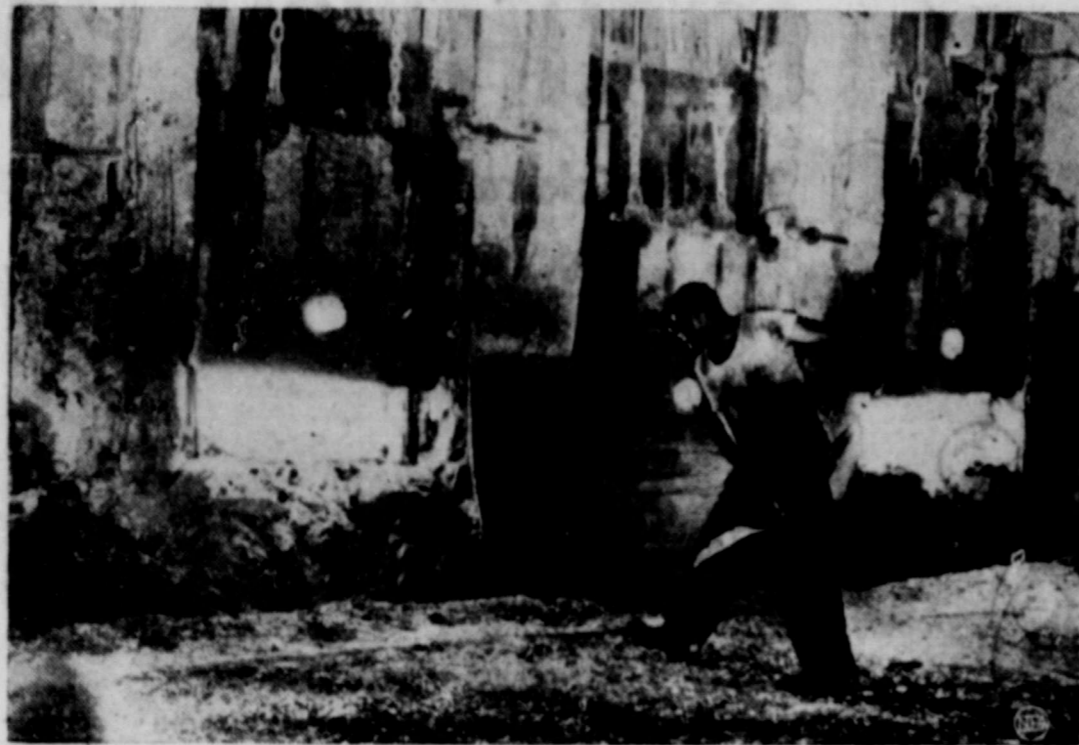
As tension mounts in the Big Steel strike threat, the Gary, Ind., works of Carnegie-Illinois Steel Corp., begin preparations for the shut down. Thomas White, a furnace helper, shovels limestone into a huge open hearth furnace at the Gary works. (NEA Telephoto.)
