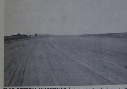
FLAT BOTTOM WATERWAY being constructed on J. W. Graham farm south of Sunnyside. Waterway will be vegetated with permanent grass and then used to dispose of runoff water from adjacent areas as well as from parallel terrace system to be installed in 1967.
