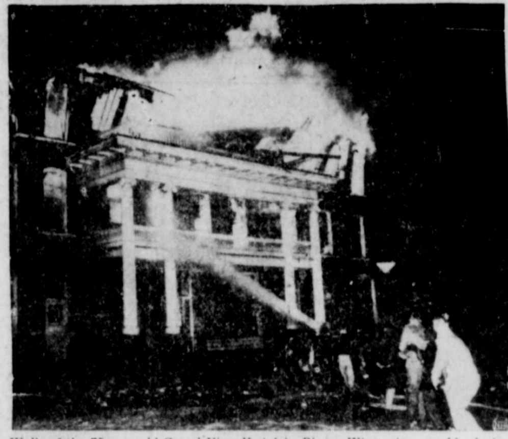
Walls of the 75-year-old Grand View Hotel in Ripon, Wisconsin, crumble during a fire which destroyed the building. Authorities feared at least five persons died in the blaze. Most of the hotel's 48 guests escaped to the street in their night clothes. (NEA Telephoto)
