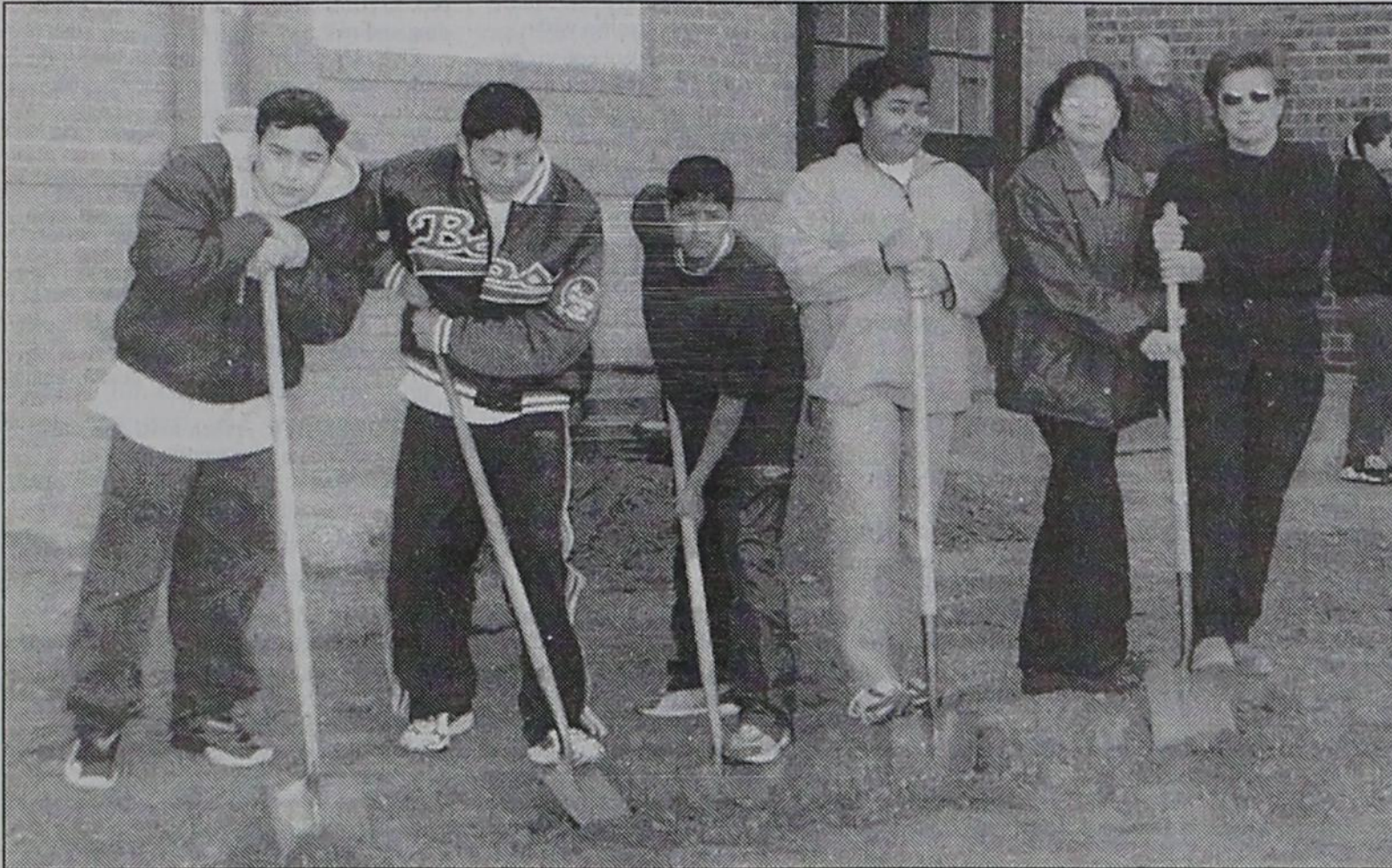
GROUNDBREAKING —Eighth grade earth science students at Dimmitt Middle School get ready to turn a shovel full of dirt to mark the "official" beginning of the construction phase of the environmental classroom project in the patio area of the school. Participating are (from left) Nicholas Cuevas, Ishmael Rodriguez, Johnny Mireles, Sarah Silva and Christy Hernandez, and their teacher Kathy Lust. The ceremony was held March 8.
