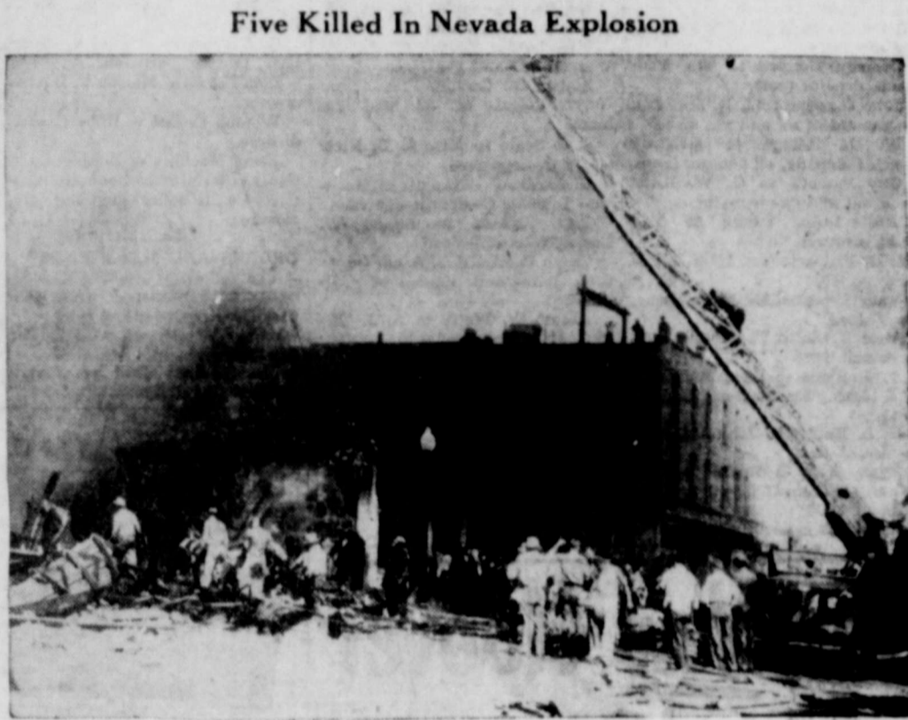
An explosion which followed a fire in Reno, Nevada, killed at least five persons and injured at least 180 others. Thirty two were seriously injured by flying glass and debris. This is a view of the building just after the explosion. Nearly half of the downtown business block was levelled by the blast. — (NEA Telephoto).
