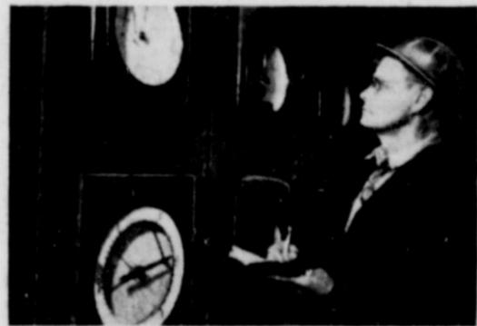
THE INDUSTRY IS EXPANDING ITS REFINING CAPACITY to meet your demand for finished petroleum products, and to increase the output of existing facilities. In 1947, Humble refineries increased their output by 12%. This picture shows the control panel at one of Baytown refinery's two catalytic cracking units; these units enable the refinery to get more finished products from each barrel of crude oil.
