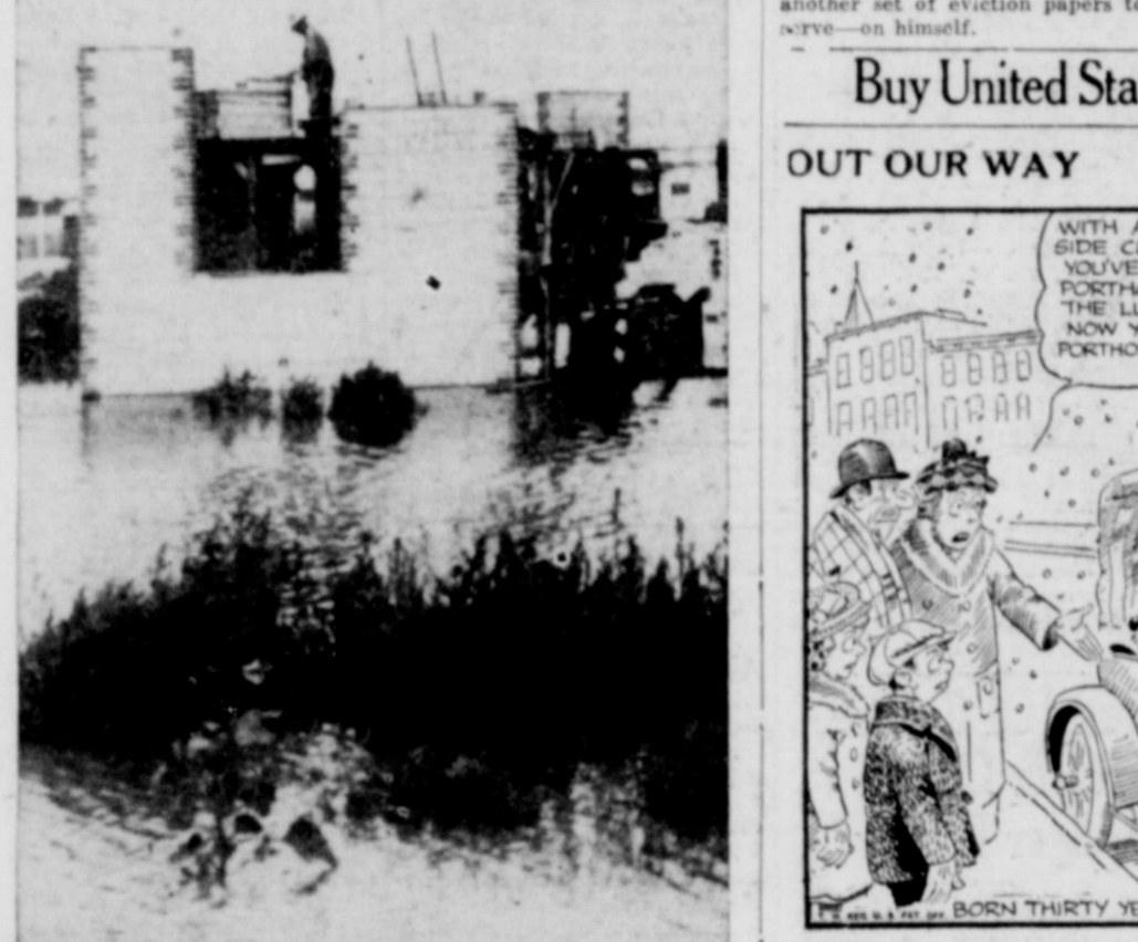
This workman isn't going to let a little thing like a raging flood keep him from laying bricks for this new house. A normally calm stream called Dry Walnut Creek, near Great Bend, Kan., became Wet Walnut Creek and flooded the surrounding area.
