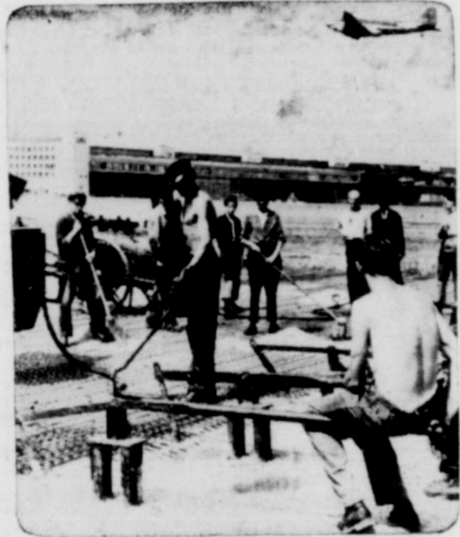
German workers put fill and tar on a temporary airstrip at the Tempelhof airdrome to repair damages caused by the great increase in traffic. The men on the right are not resting; they sit on jack handles that life the strip so tar and fill can go on bottom. — (NEA Telephoto).
