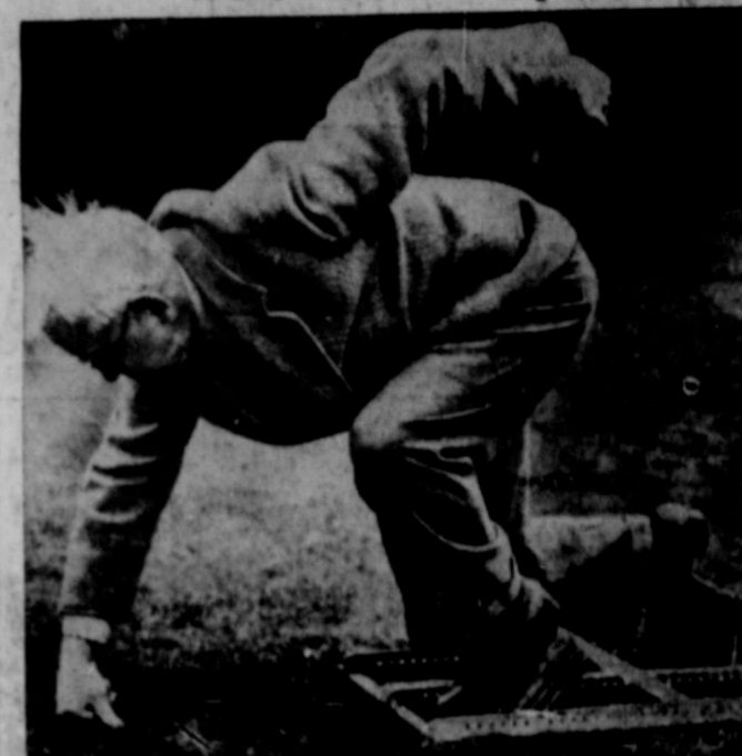
H. Hottenburg of London demonstrates the starting block he invented and his proposed starting style to help athletes in the Olympic Games this summer. The blocks can be moved backward or forward and he set at some unusual angle.
