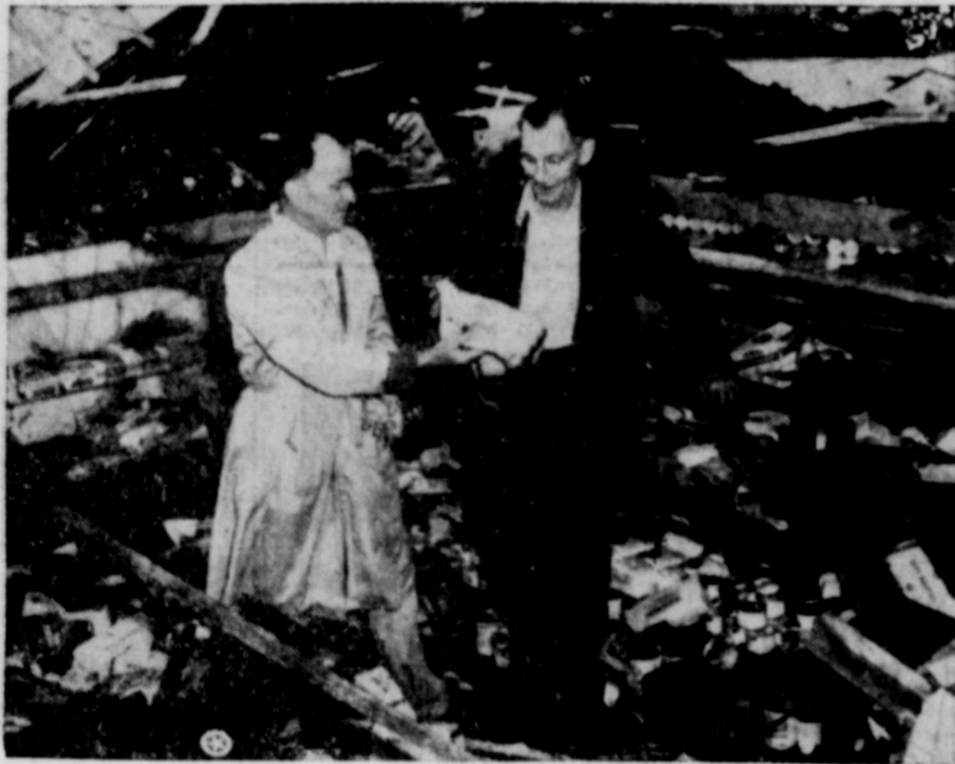
E. B. Bennett, left, and L. E. Blalock, salvage a few groceries from their McKinney, Texas, store after a tornado had completely destroyed the building. The tornado struck suddenly and damaged the community to the extent of three million dollars. Fortunately only three persons lost their lives in the disaster. (NEA Telephoto.)
