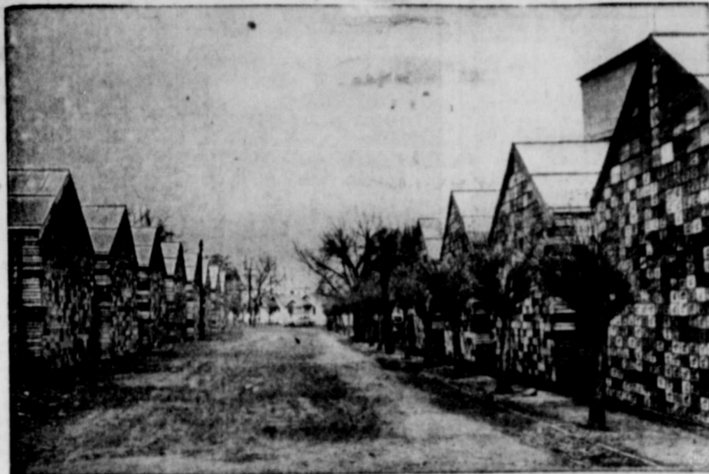
See this beautiful housing development in Yakima, Wash.? You can move in any time—if you're an apple. You're looking at Boxville, a village built entirely of tremendous stacks of apple boxes, used in harvesting and shipping Washington's huge apple crop. When not in use, they are stacked in house-like piles, with roofs to protect them against wind and rain.
