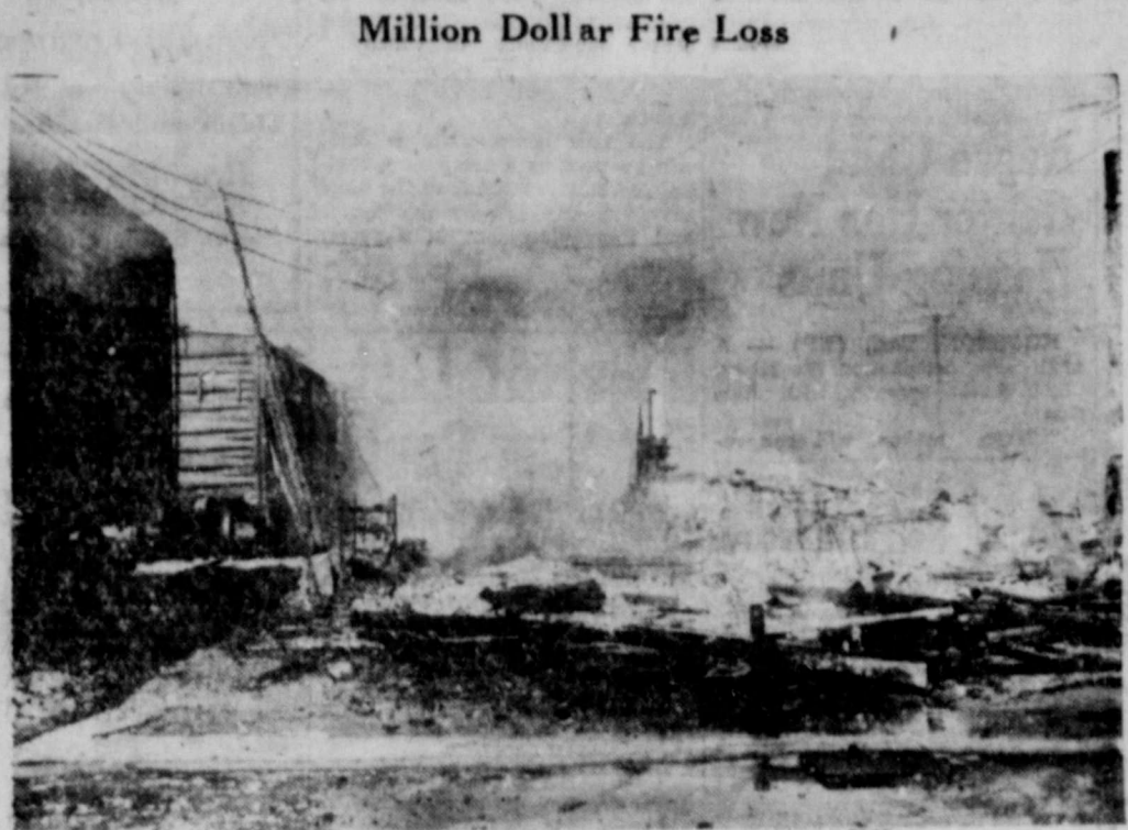
Only smoldering remains can be seen in the Texas & Pacific railroad yards just outside Shreveport, Louisiana, following a disastrous fire which swept through the yards. Fifteen rail cars were completely destroyed and 12 others damaged. The loss was estimated at nearly a million dollars. (NEA Telephoto).
