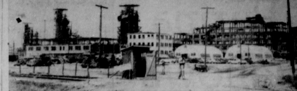
Starting on the comeback road after the Texas City, Tex., blast disaster of April 16, 1947, the Monsanto Chemical Plant is constructing a new brick building on its totally wrecked waterfront property. The flag once again flies over the charred skeleton of scientific structures, grim reminders of the shattering chain of explosions.
