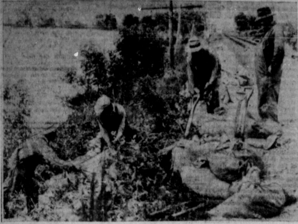
Workers sandbag the Burlington Railroad right-of-way 3 1-2 miles east of the Rulo bridge near Napier, Mo., in an effort to keep the Missouri River flood waters from weakening the embankment and undermining the rails, as new floods overflow levees along the river. (NEA Telephoto).
