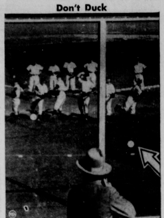
There is no need for fans sitting behind this glassed section of grandstand to duck as San Francisco Seals players hurl balls at the enclosure. The screen is three to five times stronger than ordinary glass with resistance to impact shock. Arrow points to ball bouncing off the glass.
