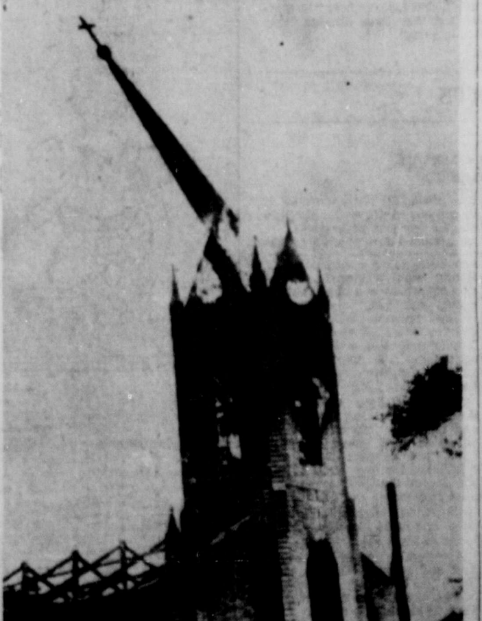
A spectacular fire in Chillicothe, Ohio, destroyed the 102-year-old St. Peter's Catholic Church, with damage estimated at a half million dollars. This dramatic shot was taken as the top of the 180-foot steeple collapsed. (NEA Telephoto.)
