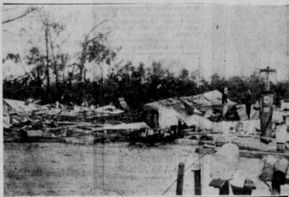
This debris is all that is left of Reed's country store at Union, Ark., when a tornado cut a path 4 miles wide through south-central Arkansas over the week-end. At left are splintered houses where nearby seven members of the E. U. Tidwell family were killed. (NEA Telephoto).
