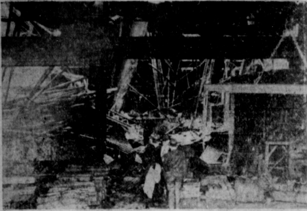
Eleven persons were injured, most of them seriously, in a furnace blast at the Lockhard Iron & Steel Company plant at McKees Rocks, Pennsylvania. Most of the injured were caught under a shower of bricks and steel. (NEA Telephoto).
