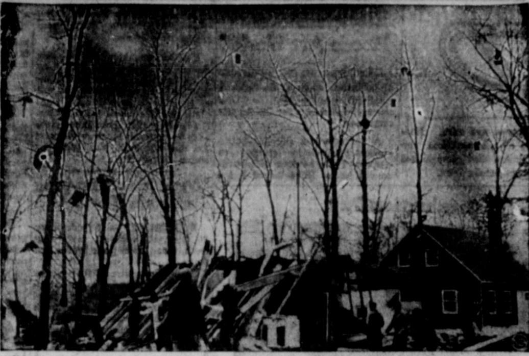
Fragments hanging from these trees resulted from an explosion of undetermined source which destroyed this new house in Albertson, N. Y. Blast injured two persons, damaged a new car.
