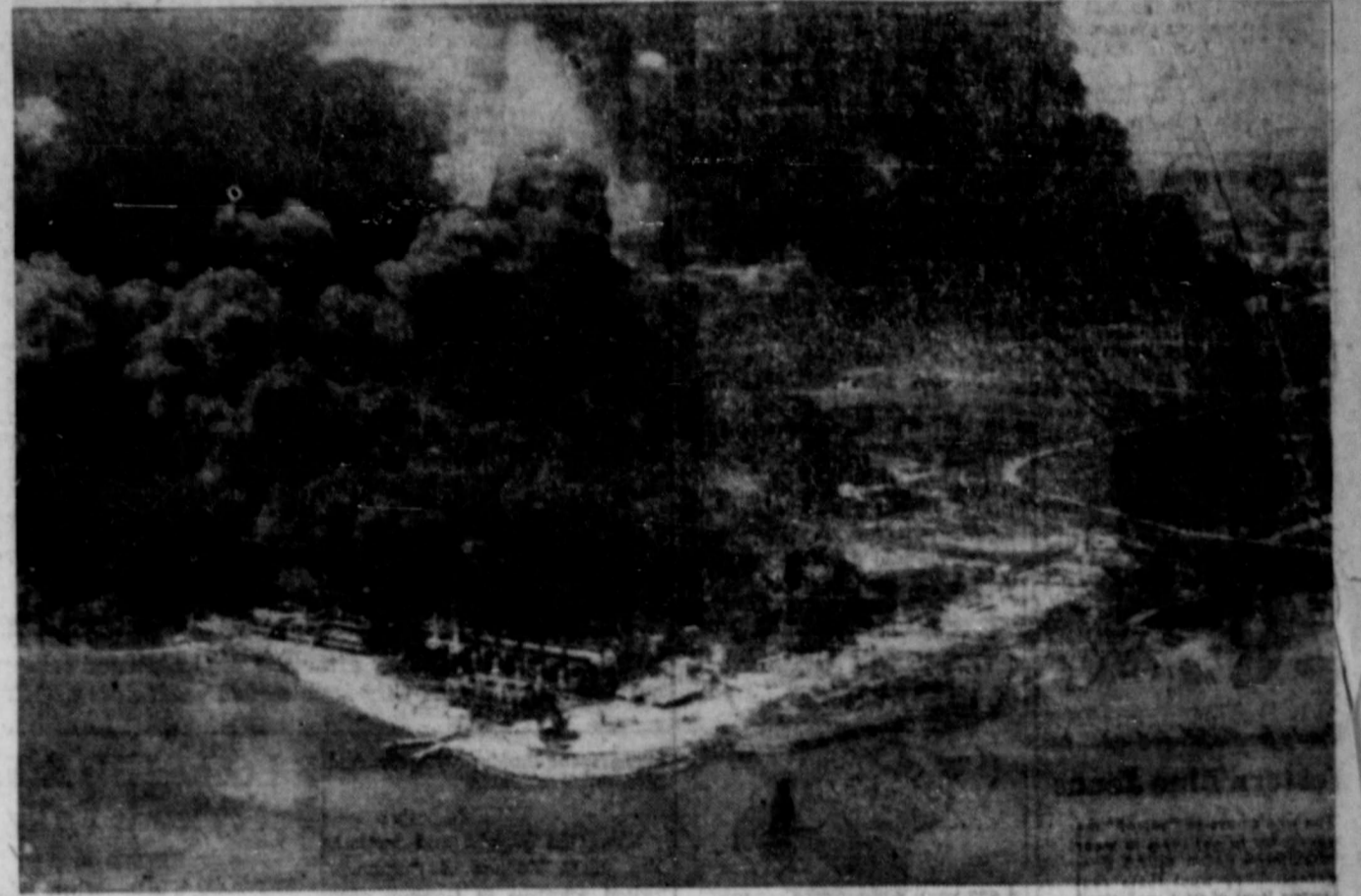
Shown is the Monsanto Chemical plant in flames after an explosion of a tank car of high octane gas set off a series of explosions and started a fire which spread to another chemical plant at Texas City resulting in reported deaths and injuries mounting into the thousands. (NEA Telephoto).
