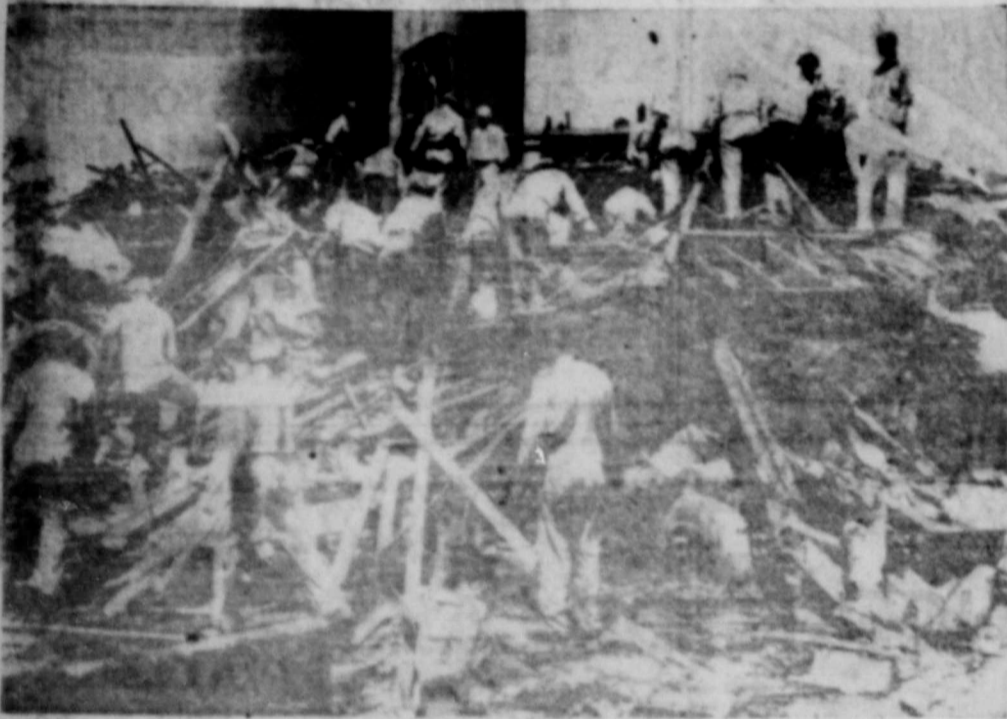
Even before the ashes cooled following the explosion and fire at the Monsanto Chemical plant, Texas City, Texas, workers were busy searching for what might remain of an estimated 40 bodies believed to have been trapped in the offices of the company. (NEA Telephoto).
