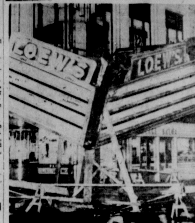
The Marquee of the Lowe's Theater collapsed under the pressure of a 60-mile-an-hour gale that roared through Indianapolis, Ind., dropping the Marquee within five-feet of the sidewalk. (NEA Telephoto).
