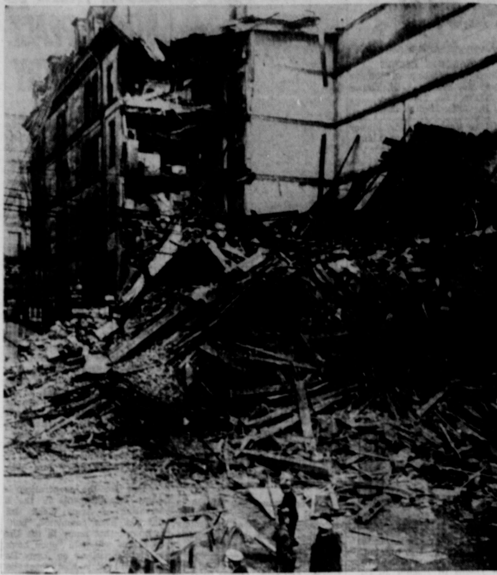
At least six persons were buried under the debris of this six-story building, which collapsed in Cincinnati, Ohio. Six other persons were injured when the building fell. Fire Chief Barney J. Houston said all the buildings in this area had been weakened by recurring Ohio River floods. (NEA Tele-photo).
