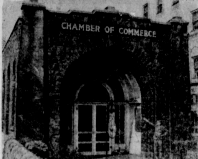
A "coal pile" unlikely to be reduced by the miners' strike is the Williamson, W. Va., Chamber of Commerce building, pictured above. Twenty feet wide, 18 feet high and 35 feet long, it is built of solid bituminous coal—60 tons of it. Coal operators and miners co-operated in erecting the building in 1933.
