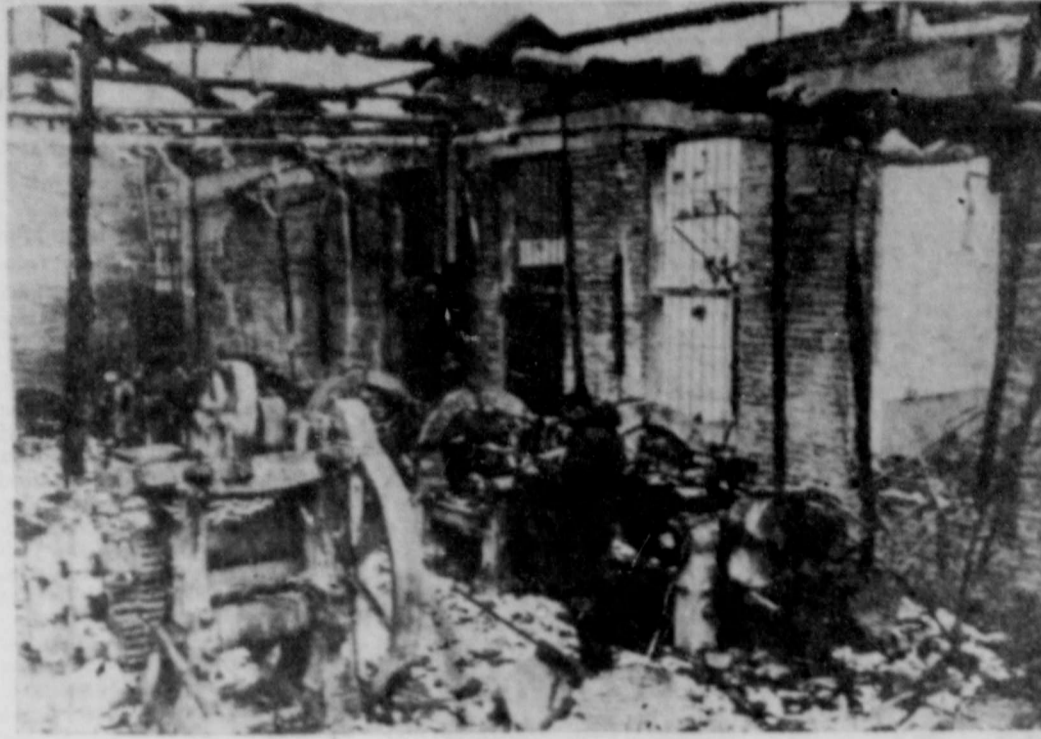
This is a general view of war wreckage of a large rubber factory in Mukden, Manchuria after the Russians had blasted holes in the walls and gutted the entire building in order to remove all the machinery. Exclusive Photo By Harlow M. Church from NEA Telephoto.
