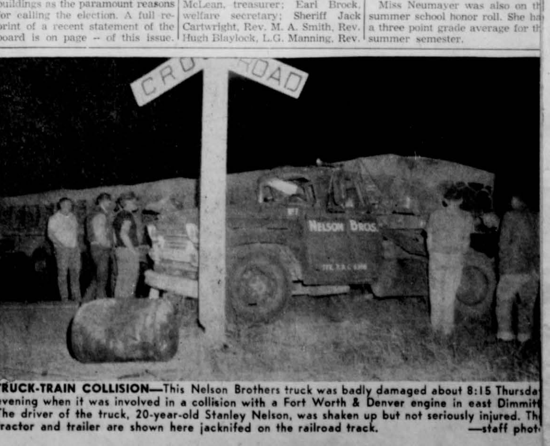
TRUCK-TRAIN COLLISION—This Nelson Brothers truck was badly damaged about 8:15 Thursday evening when it was involved in a collision with a Fort Worth & Denver engine in east Dimmitt. The driver of the truck, 20-year-old Stanley Nelson, was shaken up but not seriously injured. The tractor and trailer are shown here jackknifed on the railroad track. —staff photo
