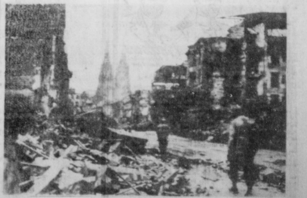
Troops of the 3rd armored division, 1st Army, advance through the ruins of Cologne, Germany. Twin spires of the famous cathedral only five blocks away, are undamaged. (Signal Corps radiotelephone from NEA TELEPHONE)
