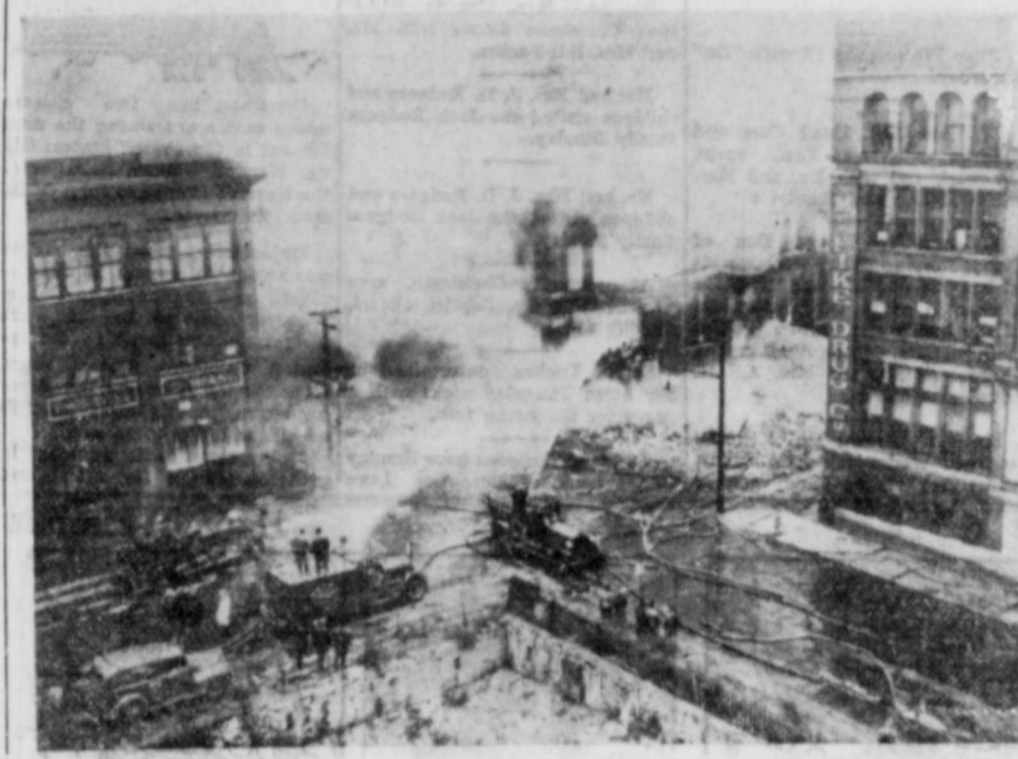
Three buildings at Seventh and Central streets, Kansas City, Mo., blaze in an all-alarm fire which destroyed one building and caused an estimated damage of $2,390,000 in the immediate area. Twenty-five companies struggled the tremendous blaze for six and one-half hours before it finally was brought under control. (NEA Telephoto.)
