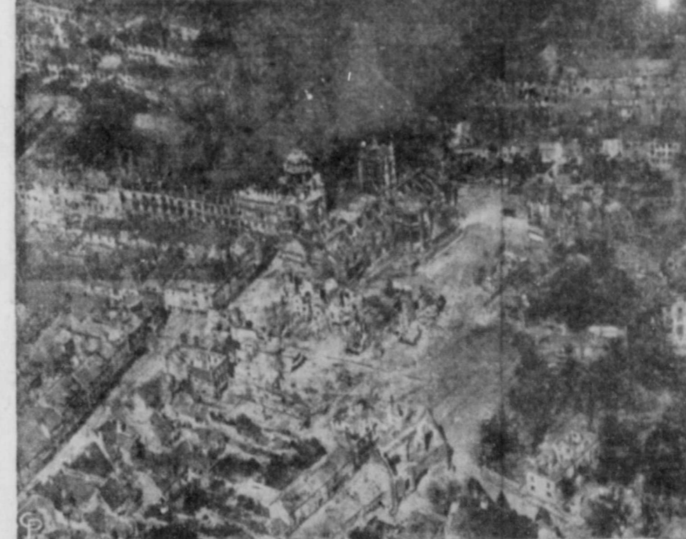
THE TOWN OF ARGENTAN, FRANCE, resembles a scene of ancient ruins in this air view showing damage caused by American artillery and bombing attacks in driving the Nazis from the town. This is an official United States Army Signal Corps photo. (International Soundphoto)
