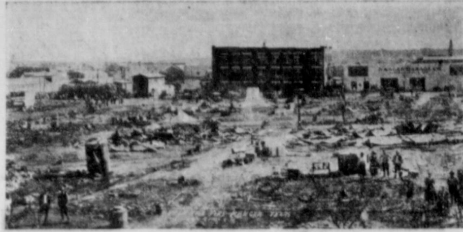
The picture above shows the ruins of two square blocks of Ranger's business district after a disastrous fire swept it on April 6-7, 1919. The fire ravaged the two blocks between Rusk and Marston streets, burning everything from Main back over to Walnut street. Damage was estimated at $850,000 and there was very little insurance carried on the burned properties. One life was lost in the fire and many were injured. The brick building shown in the picture is the famous McCleskey hotel, which later was destroyed by fire which took the lives of several people.
