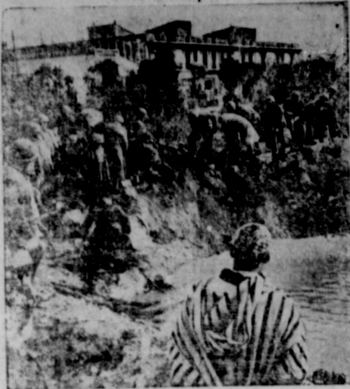
Light picks and shovels American soldiers fill a crater resulting from a land air raid on Cambes. As the hole is being filled, loose earth is being blown off by a broken main.
