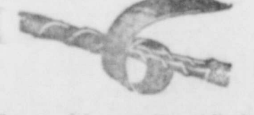
Then tape wires together. Adhesive tape cures and cracks very quickly.
