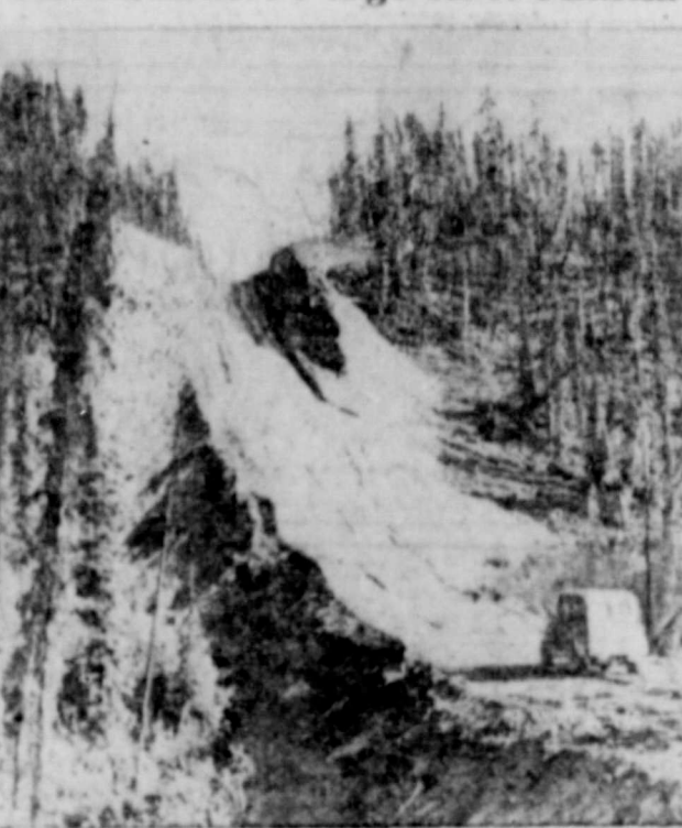
Workers on the new "Alcan" military road across Canada to connect the U. S. with Alaska are making rapid progress as they equalize topography by cutting through hilltop such as that shown above.
