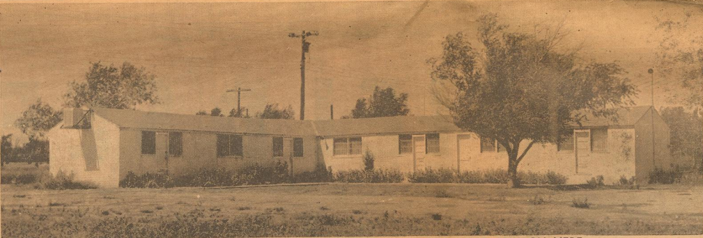
NOW BETHEL MISSION, BUT SOON TO BE LEE STREET BAPTIST CHURCH HERE
