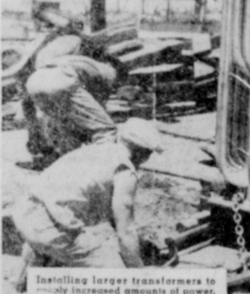
Installing larger transformers to supply increased amounts of power.
