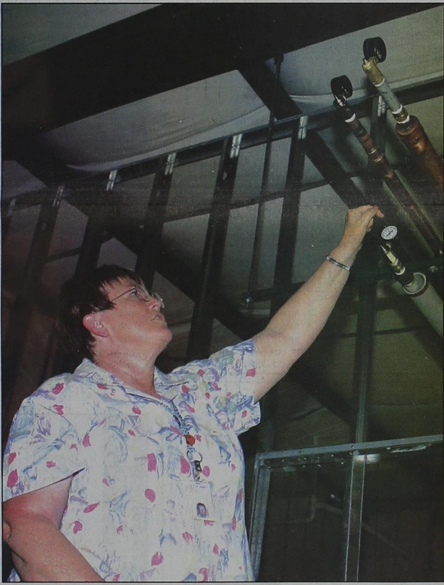
KAREN HUTSON , the city's code enforcement officer, checks out the pressure valves for some of the plumbing inside the new, state-of-the-art Pioneer Dairy Lab.
