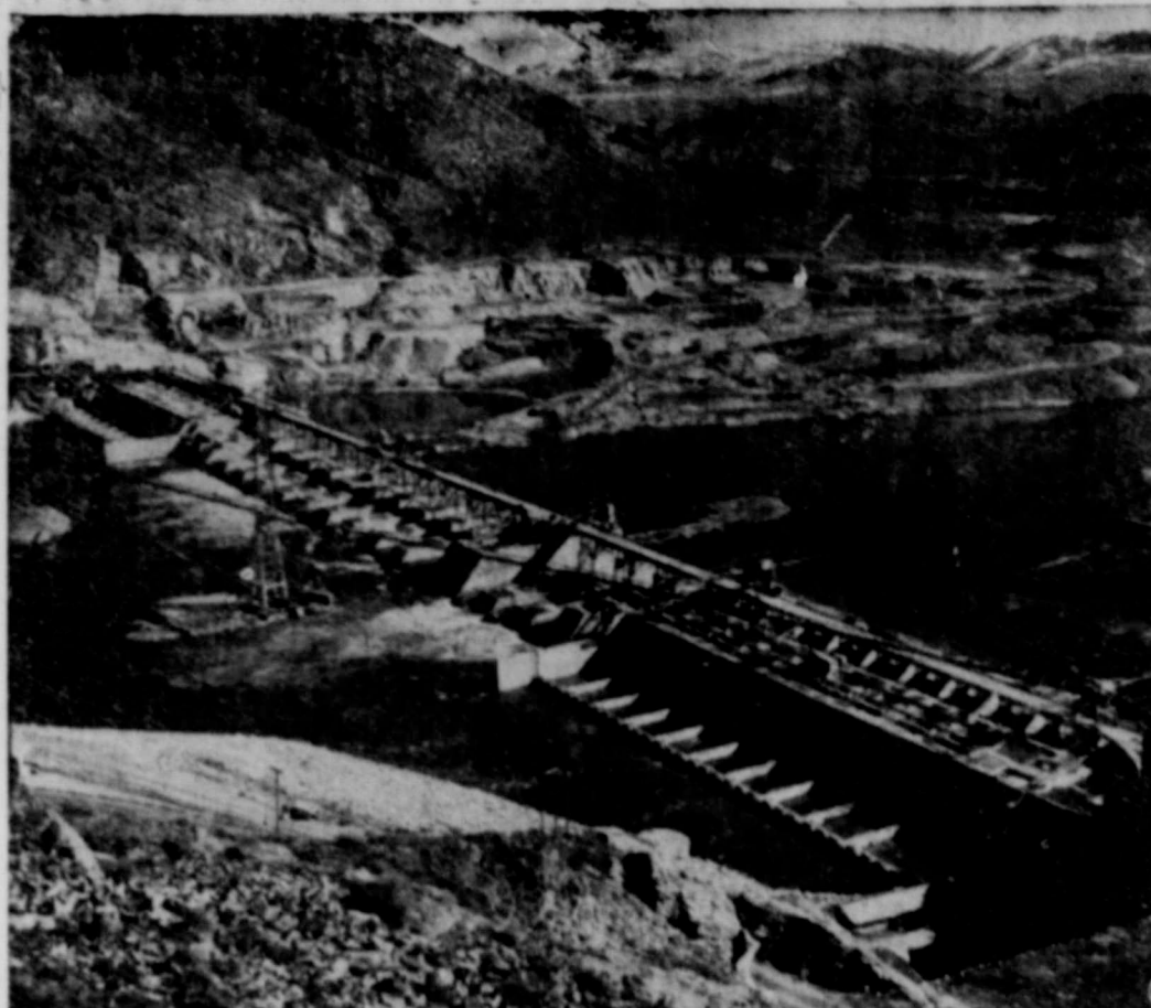
Airview shows the huge bulk of Grand Coulee Dam—a barrier three-quarters of a mile long across the Columbia River.
