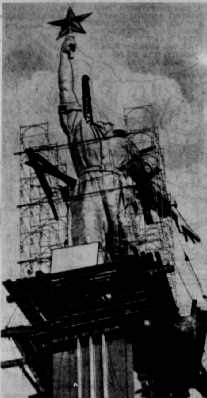
Of gleaming stainless steel—79 feet from toe to the tip of the 12-foot star it bears aloft—weighing 30 tons—dominant figure of the New York World's Fair skyline—dubbed "Big Joe," but officially, "The Worker." Off comes Joe's thousand-pound head, as workmen begin dismemberment of the gigantic statue surmounting the Soviet Pavilion. The parts will be shipped back to Russia to be reassembled.
