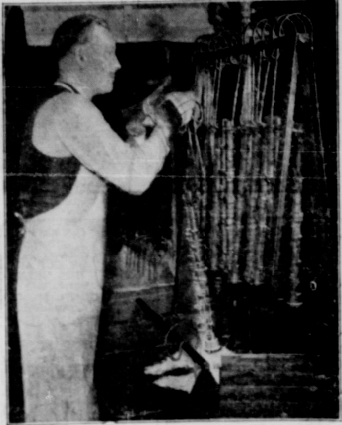
Hudson has adopted a new method of treating the cam surfaces on the camshaft which eliminates the harmful effects of the break-in period according to Hudson engineers. Photo shows the new treatment known as Grand-Dizing which consists of a formula bath which causes the surface of the cam to absorb and hold oil, thus adding greatly to the life of the cam.
