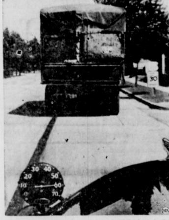
No matter how hard he argues, the driver of the truck in the above picture won't convince a judge he wasn't traveling 60 miles on a 30-mile speed limit highway. A camera on the windshield of the car following the truck photographed simult the truck, a speedometer (registering 60 miles an hour) attached to the left front fender of the trailing auto, and the 30-mile speed limit sign. It's a new device in the war on speeders exhibited at the National Safety Council Congress in Chicago.
