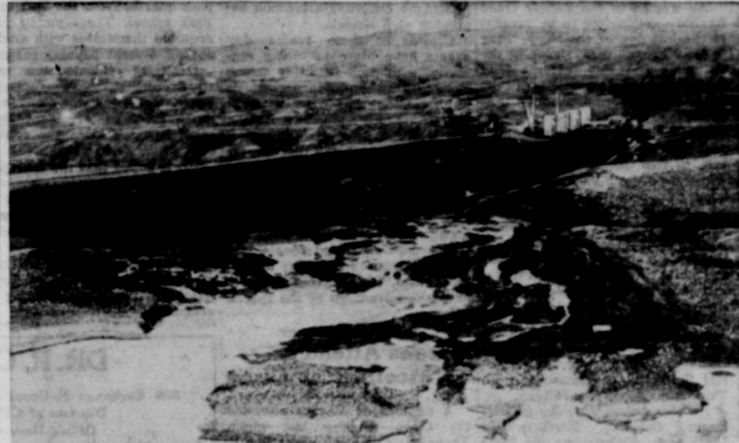
A tremendous earth slide which carried away part of the upstream face of Fort Peck Dam, near Glasgow, Mont., and which probably killed eight men, is seen in the center of the above air photo. The PWA project is the largest earth-fill dam in the world, and damage is expected to cost $2,000,000 to repair, though the 180-mile lake backed up in the Missouri behind the dam is believed safely held by the main sections of the dam, which stood firm. Cause of the slide had not yet been determined by Army engineers in charge.
