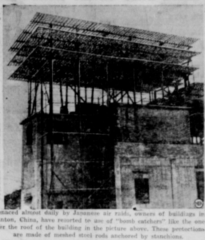
Menaced almost daily by Japanese air raids, owners of buildings in Canton, China, have resorted to use of "bomb catchers" like the one over the roof of the building in the picture above. These protections are made of meshed steel rods anchored by stanchions.
