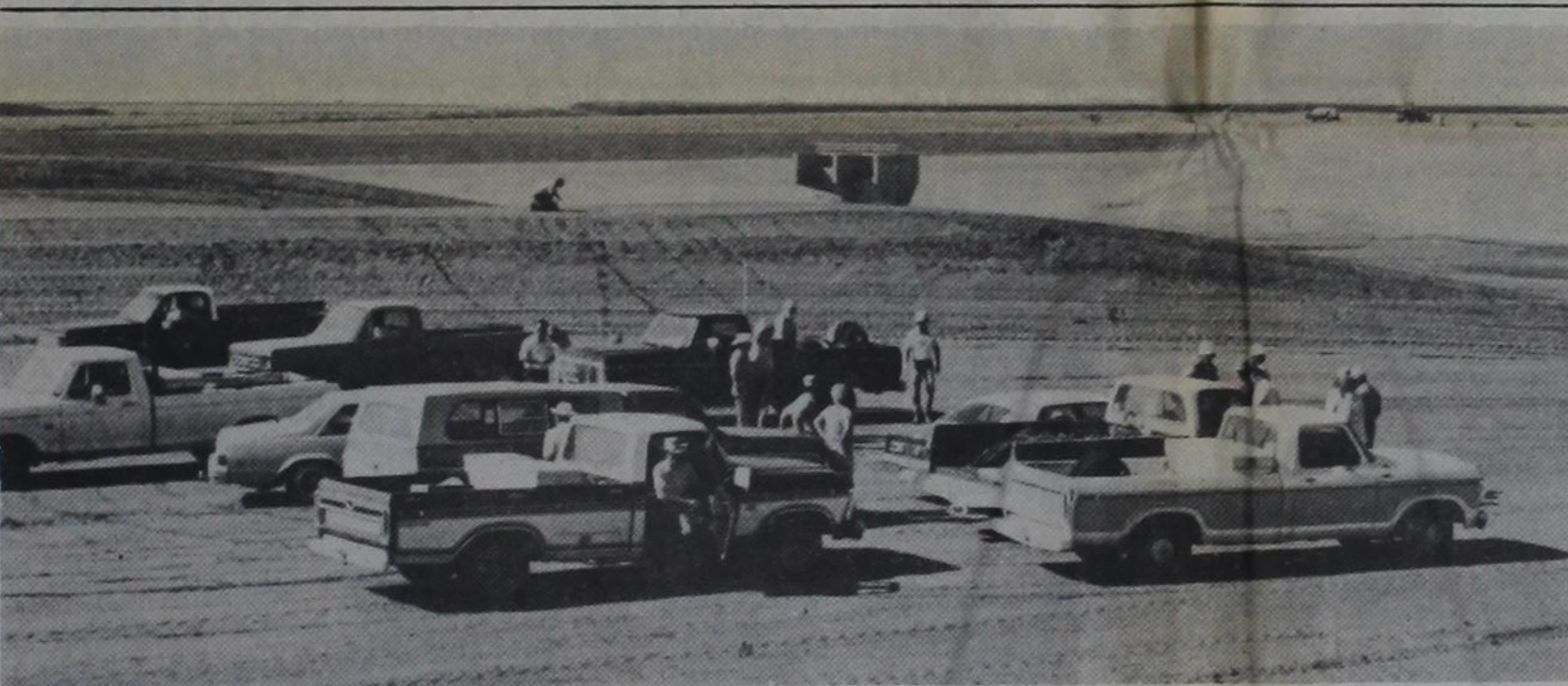
DRY RUN —County and Soil Conservation Service officials park on the emergency spillway of the Lower Running Water Draw Watershed Reservoir east of Sunnyside during an inspection tour of the project Tuesday morning. In background is the earth-and-concrete dam with the floodgate structure in the center. Light-colored slope in right background is the south
